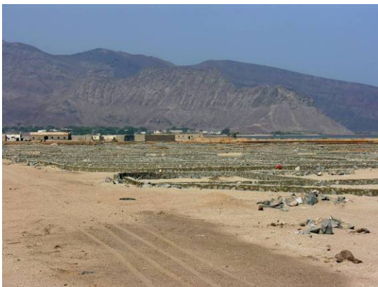
Foundations for 2,600 new houses beside Al-Farsi village
