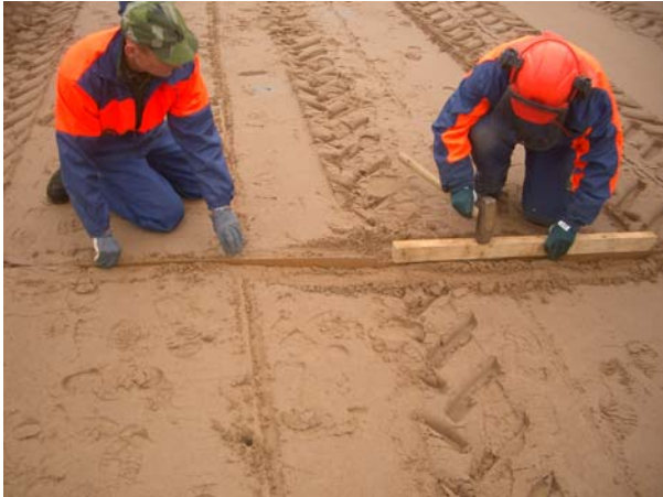
Fixture and fitting of the fibreboard into the ground. © CCMAT
