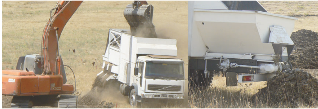
Sifter loaded by excavator
