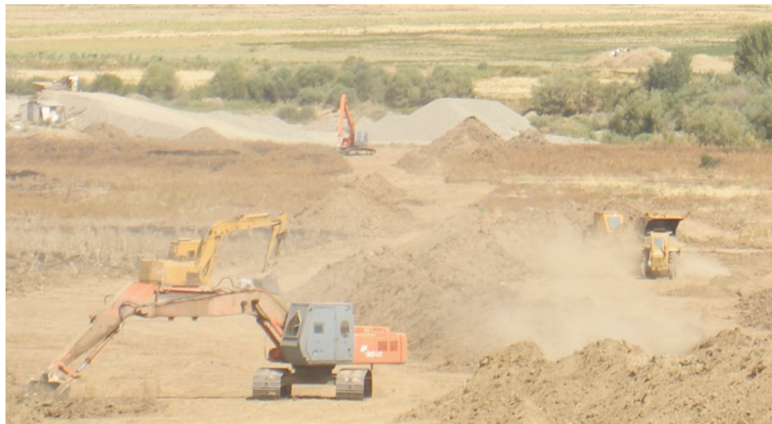
Sifter in mine clearance area
