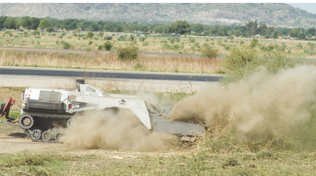
DIGGER 2 | Operating along runway
