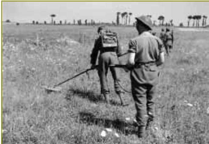
Figure 2. R.E.s (Royal Engineers) searching for mines with mine detectors before a bypass road is constructed around the French village of Douvres-la-Delivrande, 1945.
