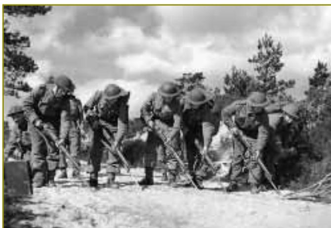
Figure 1. British Army mine clearance of a road in 1945. Soldiers using their rifles and bayonets to detect mines. This is called the ‘prodding’ method and the ground is prodded with the bayonets to clear a lane the width of six or seven men. White tapes are used to mark the boundary as it is cleared.
