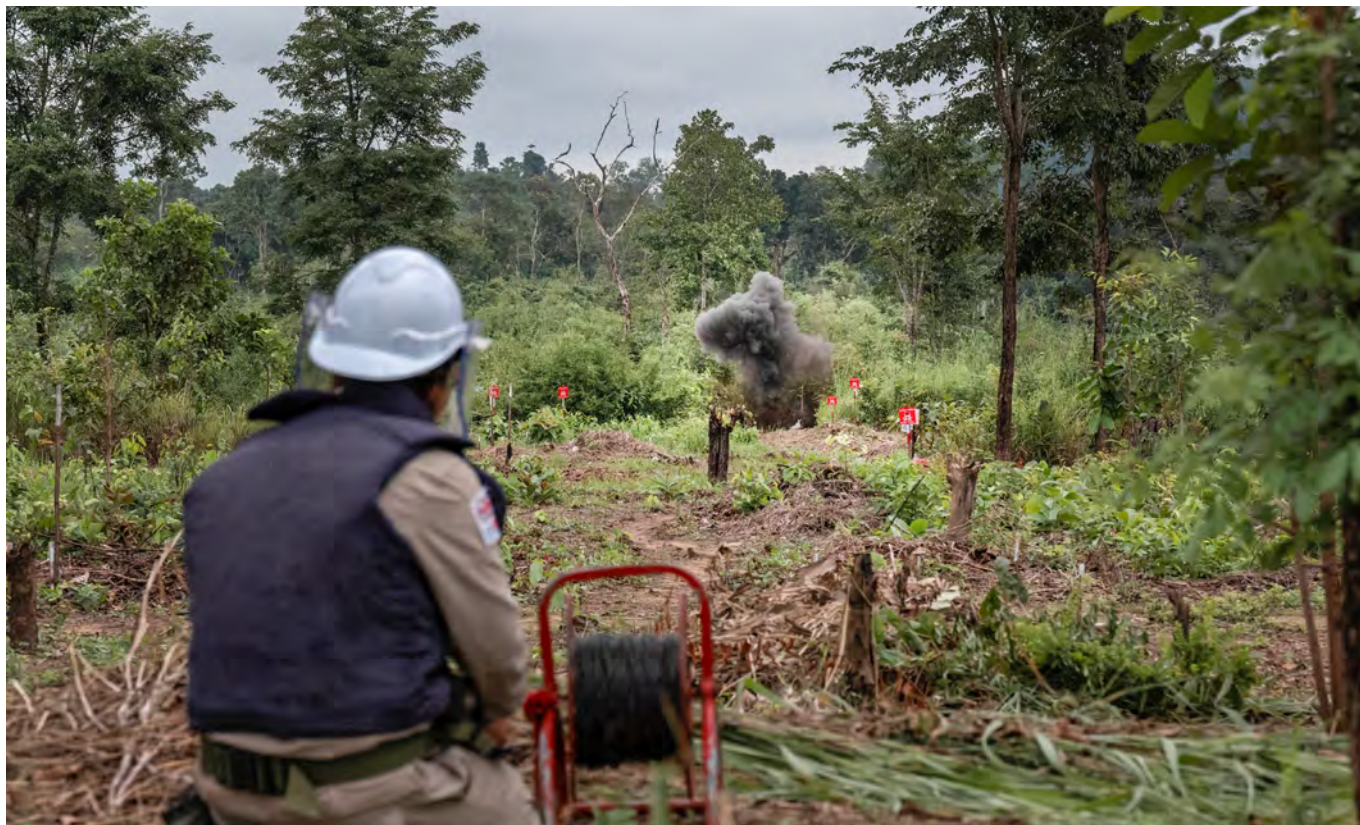
Demolitions commonly takes place in situ where explosive ordnance items are found. Demolitions of not-safe to move items in urban areas carry additional risks to already damaged or vulnerable structures. Picture: A demolition of antipersonnel landmine in an open field in Cambodia. © MAG (Mines Advisory Group) 2022
