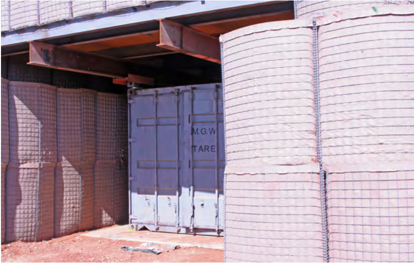
Figure 20 – Shipping Container Based Magazine with Overhead Protection. 100)
