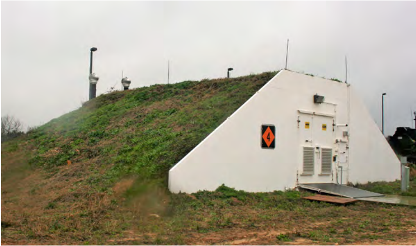
Figure 25 – Pre-Fabricated Metal Earth Covered Magazine - As Built. 105)
