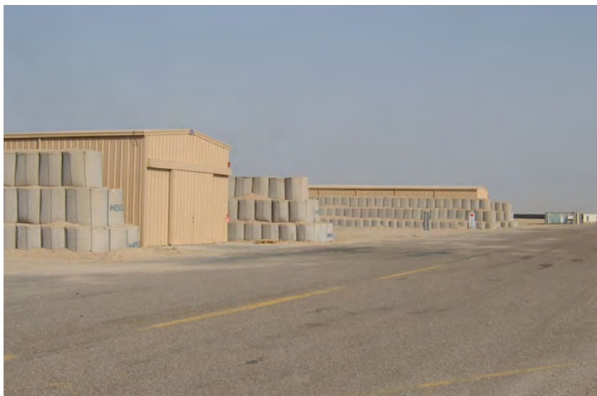
Figure 22 – Barricaded Light Walled Frangible Ammunition Storage Solution. 102)
