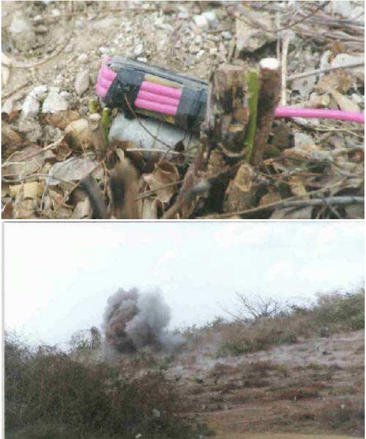
Figure 2.8: Elimination of small UXO by blast-in-situ. .
