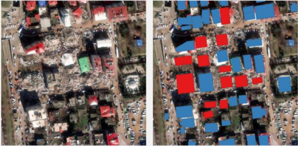
Figure 7: A set of nine destroyed 5-story apartment buildings in downtown Islahiye. Maxar Technologies, Feb 7th.
